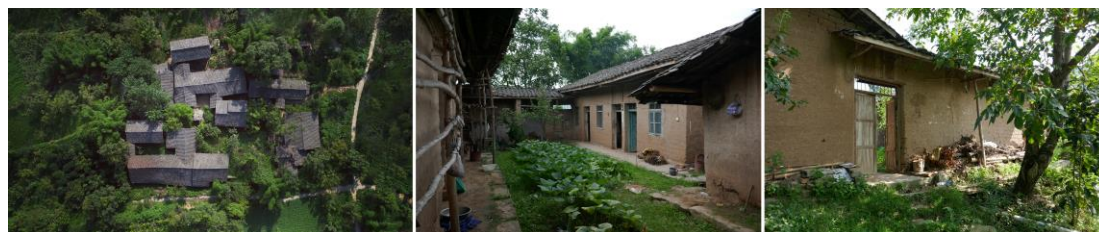
Figure 1. Bird's eye view of Li's house, The inner courtyard on the south side of Li's house, Outside the south side of Li's house Source by author [2017]
