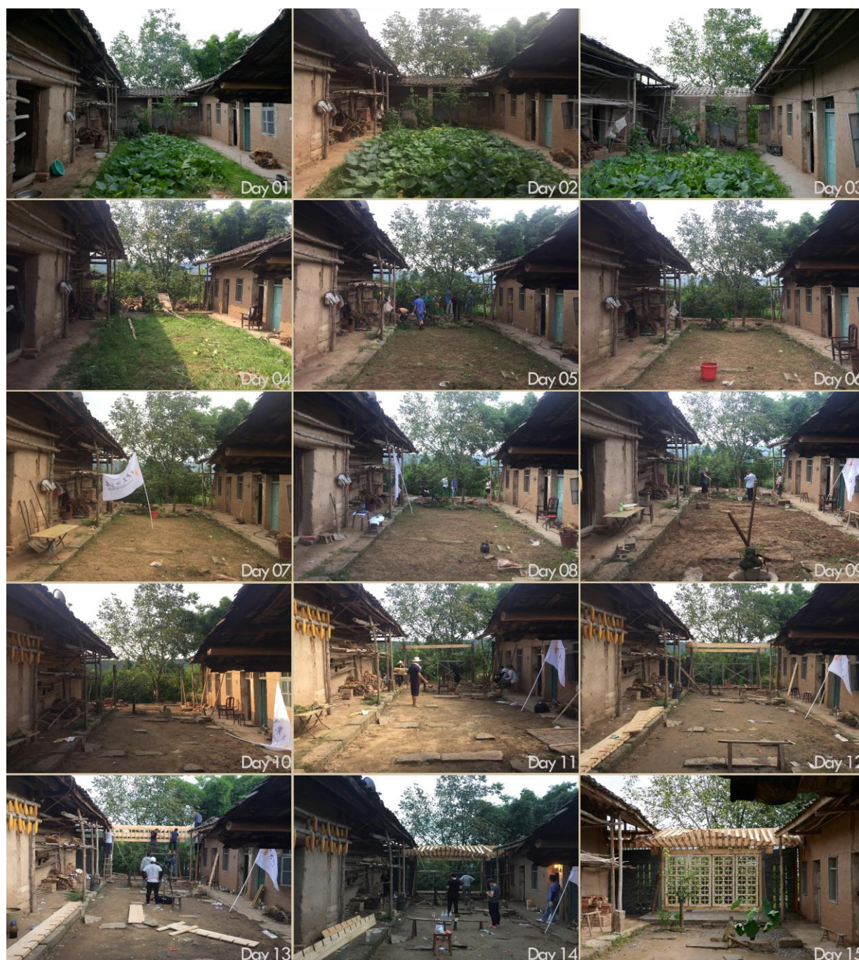
Figure 6. Fixed-point photography of the 15-day construction process Source by author [2017]
