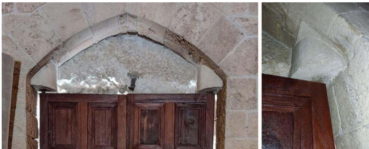
Figure 3. The upper stone gudgeons of the southern door of Saint John in Jubayl [Dania Keyrouz, 2021].
