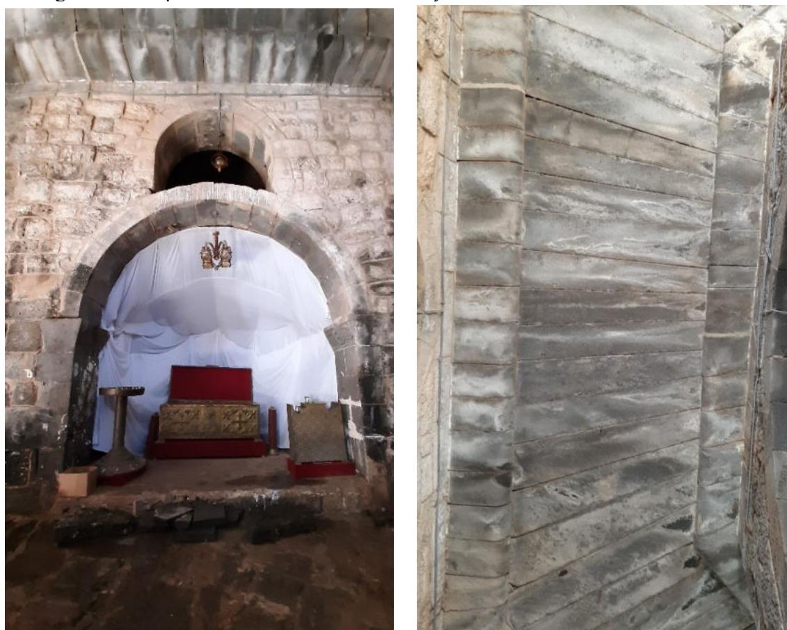
Figure 15: The right picture illustrates exedra . The left picture shows the roof which is a corbelled stone slab of the south aisle. Photo by researcher in 2019.
