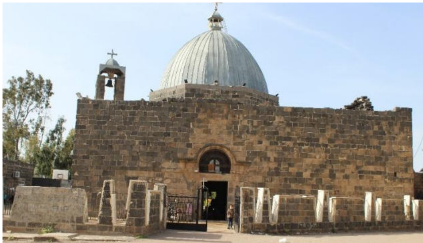
Figure 17: Southern façade of the church. Photo by researcher in 2019.
