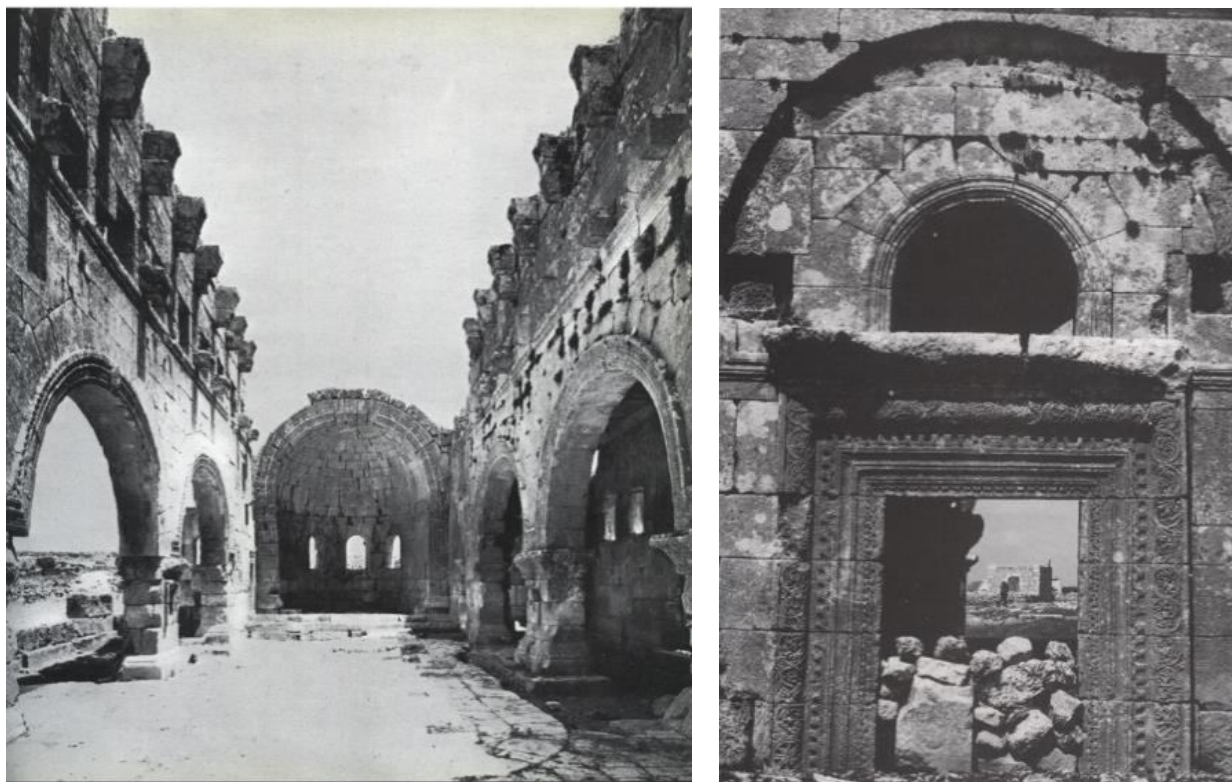
Figure 19: Interior viewing East: central nave, piers and wide arches. (Mango, Architecture Byzantine , 1979, p. 80). This picture presents the western entrance of Qalb loze church (for men). (Peña, 1997, p. 88).
