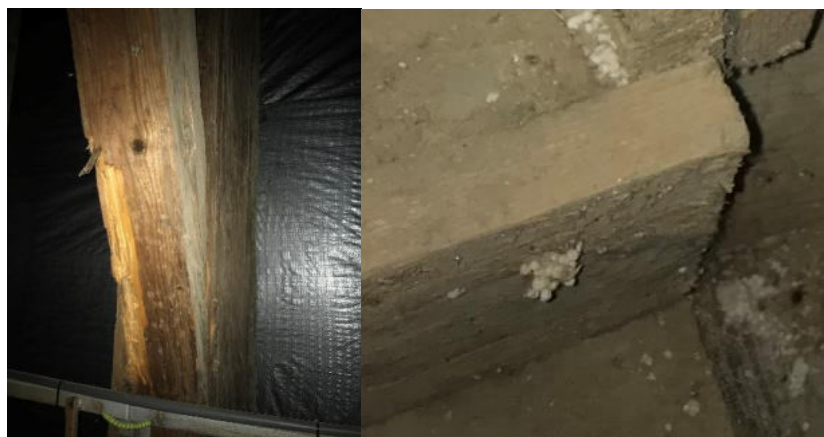
Figure 5: Wood defects: a – surface crack, b – fungal growth
